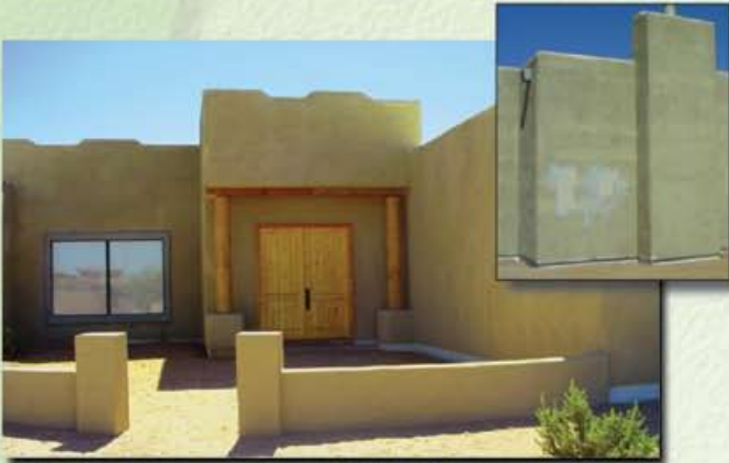
ORO Coatings repairs existing hard coat stucco
