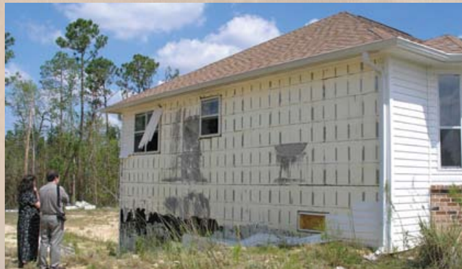
All Photos Courtesy of American PolySteel
