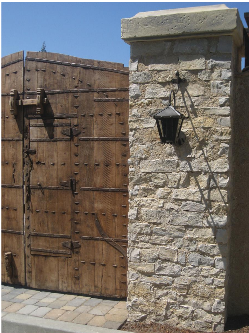
The stone veneer pieces range in size from 2 and 6 inches in height.
