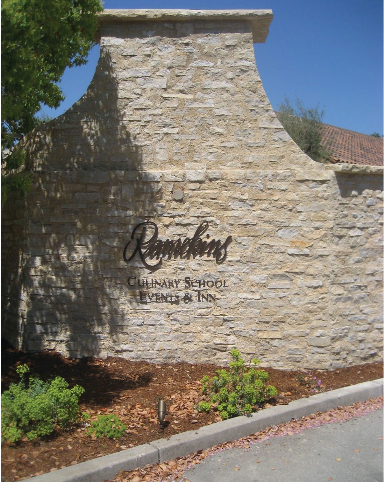
Stucco was placed over the stone and joints to give the exterior architecture the feel of a French chateau.
